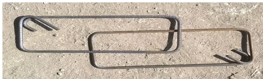
Photo No.3: Reinforcement for Beam Design
