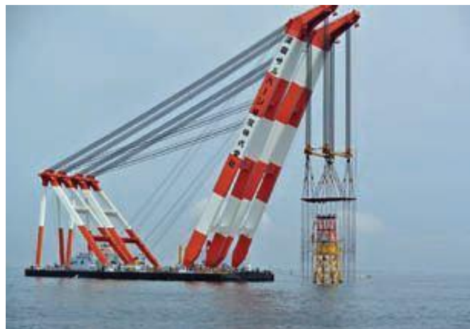
Fig. 1. Offshore support structure installation by crane lifting and down positioning
