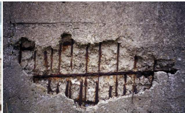
Fig 1.3 Spalling of concrete
