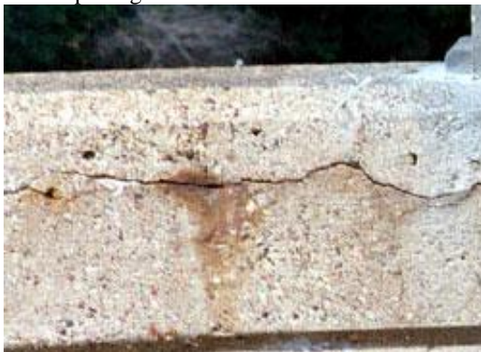
Fig 1.2 Cracking of concrete
