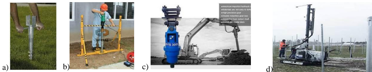
Fig.2: Method of screwing
