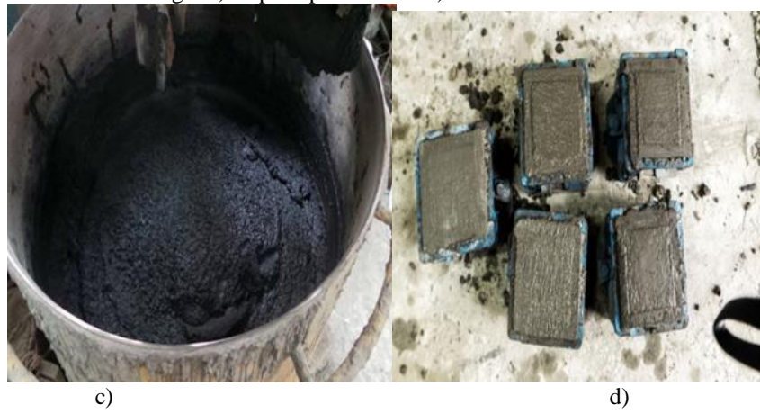
Fig 2. c) Blending of fibres in concrete mix d) Concrete poured in
