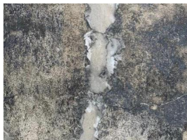
Figure 12: Dry Packing
