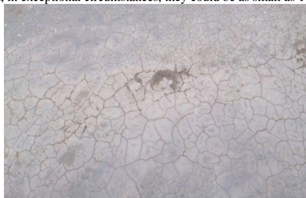
Figure 6: Concrete crazing [17].
