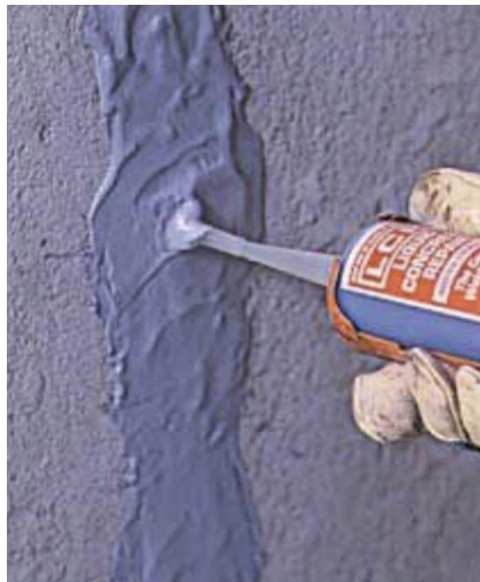
Figure 8: Epoxy Injection Method.
