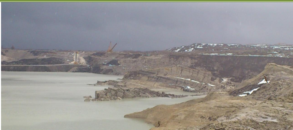
Figure 3: Launched marl blocks from the south side and the formation of an artificial accumulation in the Gacko coal mine
