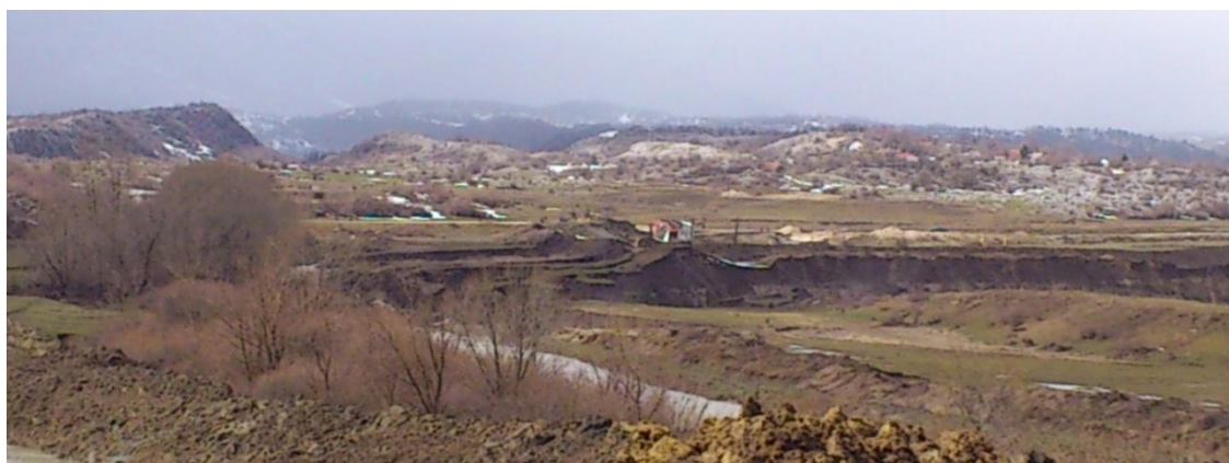
Figure 4: Landslide on the western side of the surface mine (Gojković stream zone)
