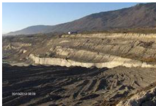
Figure 9: Dredging on slopes
