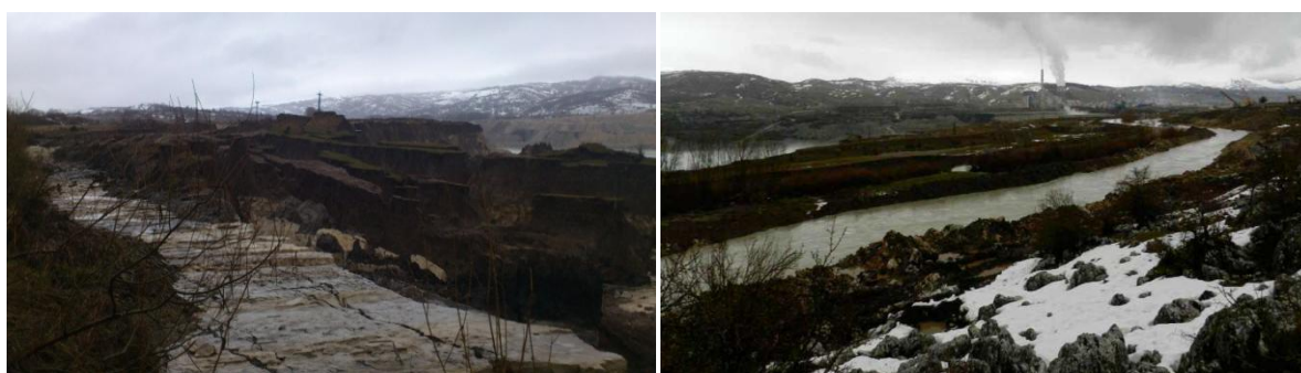
Pictures 1 and 2: Movement of blocks from the south side of the surface mine (zone of river penetration into the mine)
