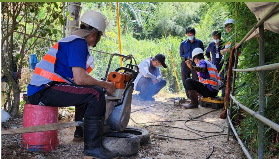
Fig. 3-3-7. Small portable winch used as an auxiliary winch.
