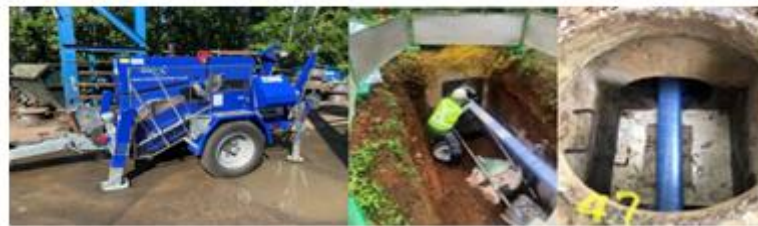
Fig.2.3 10-ton pulling winch and liner insertion
