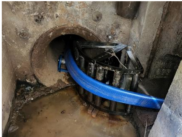
Fig. 3-3-3. Roller set comprising rollers lined up in a curve.
